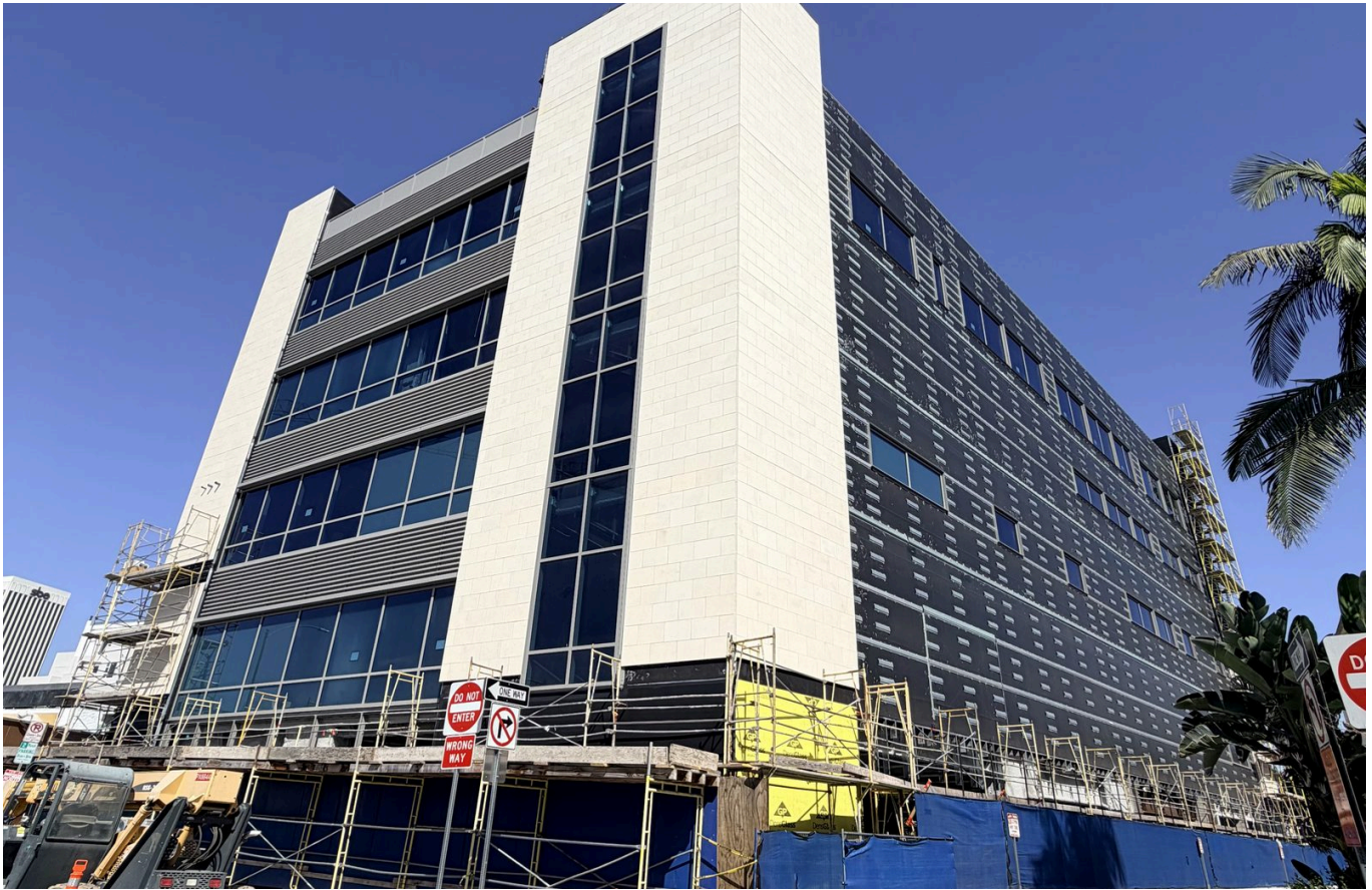
EXHIBIT 5. SOUTHWEST ELEVATION. APRIL 2026.
