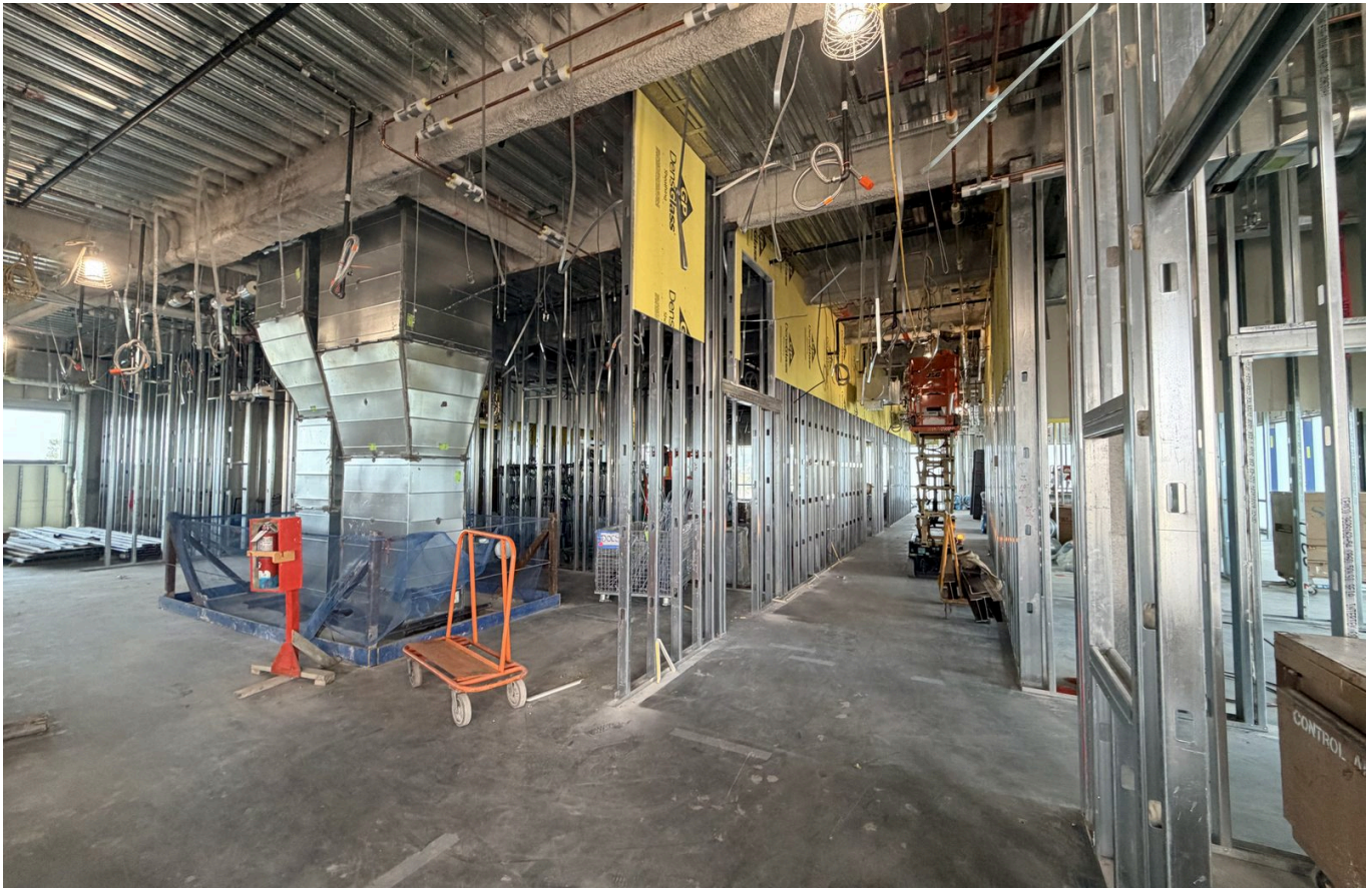
EXHIBIT 4. THIRD-FLOOR CORRIDOR. APRIL 2026.
