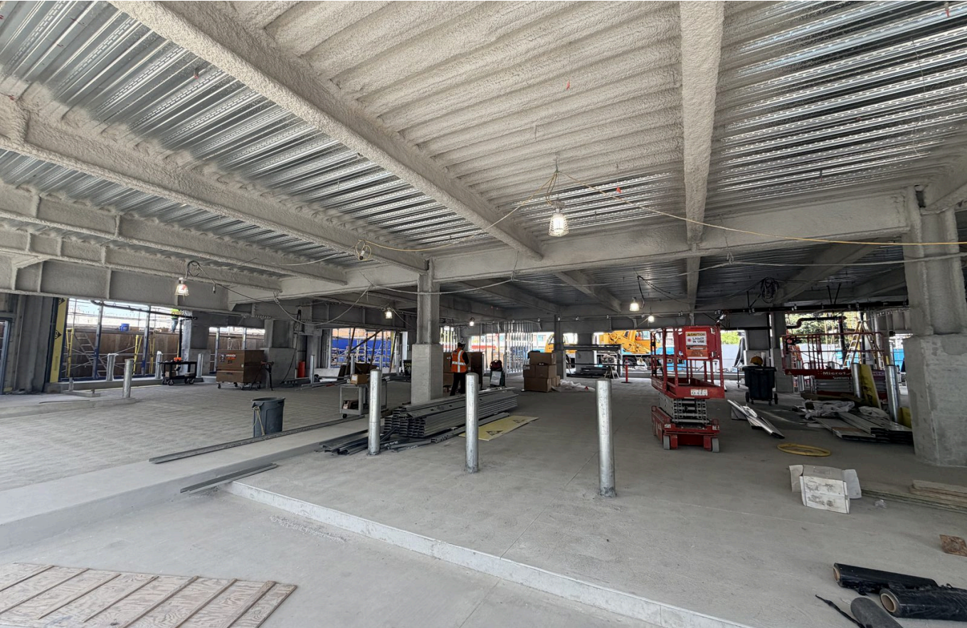
EXHIBIT 2. GROUND-FLOOR SHELL. APRIL 2026.
