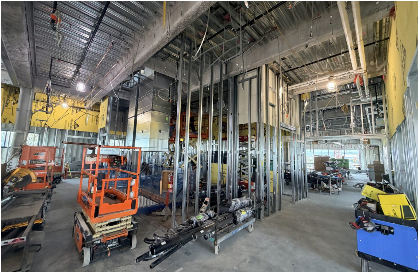
EXHIBIT 3. FOURTH-FLOOR FRAMING WITH OVERHEAD ROUGH-IN IN PROGRESS. APRIL 2026.
